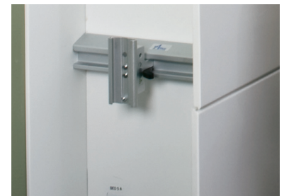
Lap jointed removable panels
