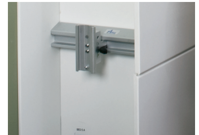
Lap jointed removable panels
